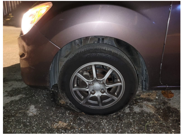
Fig. 2: Example of road with potholes.
