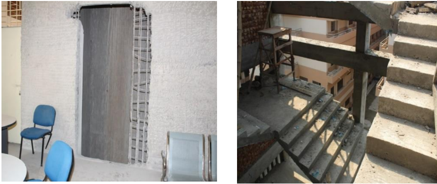
Fig. 5: Unprotected lift core and staircase
