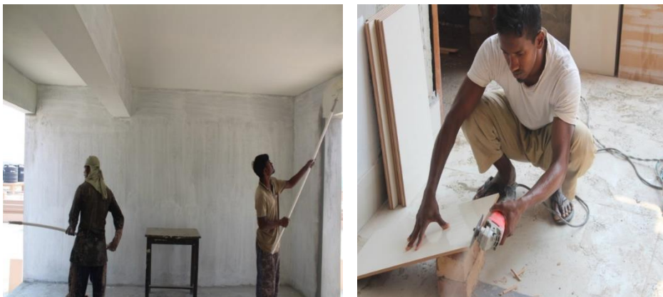
Fig. 3: Labour working without hand gloves, eye protective tools during painting & cutting.
