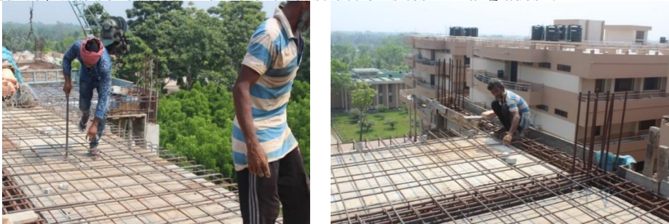
Fig. 1: Labor working without any fall protective guardrail system.
