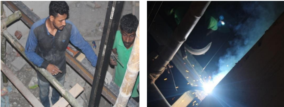
Fig 7. Workers working without hand gloves, helmets and poor eye protection during welding in lift installation.
