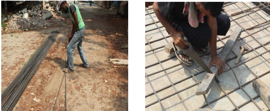
Fig. 4: Labor working without protective measures during bending rod & cutting wood
