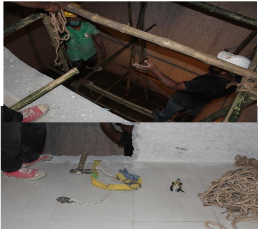
Fig. 6: Working environment without fall protective system and safety belt was provided which was not used.
