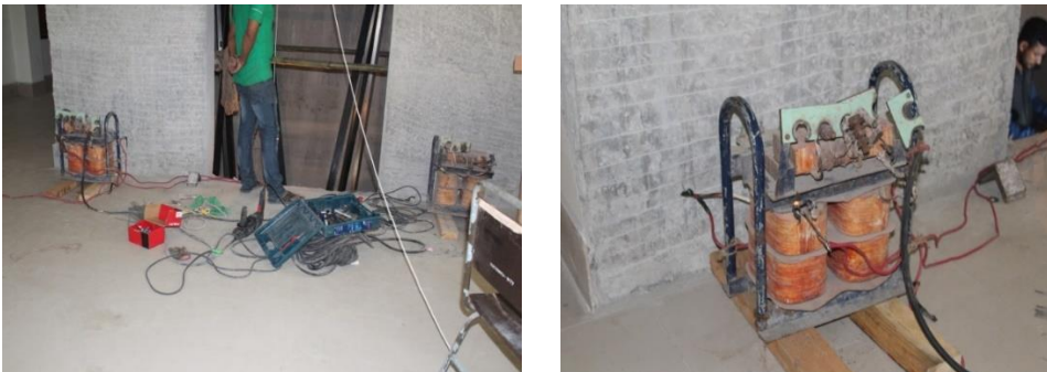
Fig. 8: Electrical wires and equipment are kept in hazardous condition.
