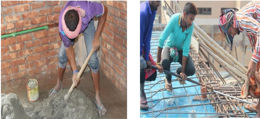
Fig. 2: Worker working without safety boots, hand gloves, head protection.
